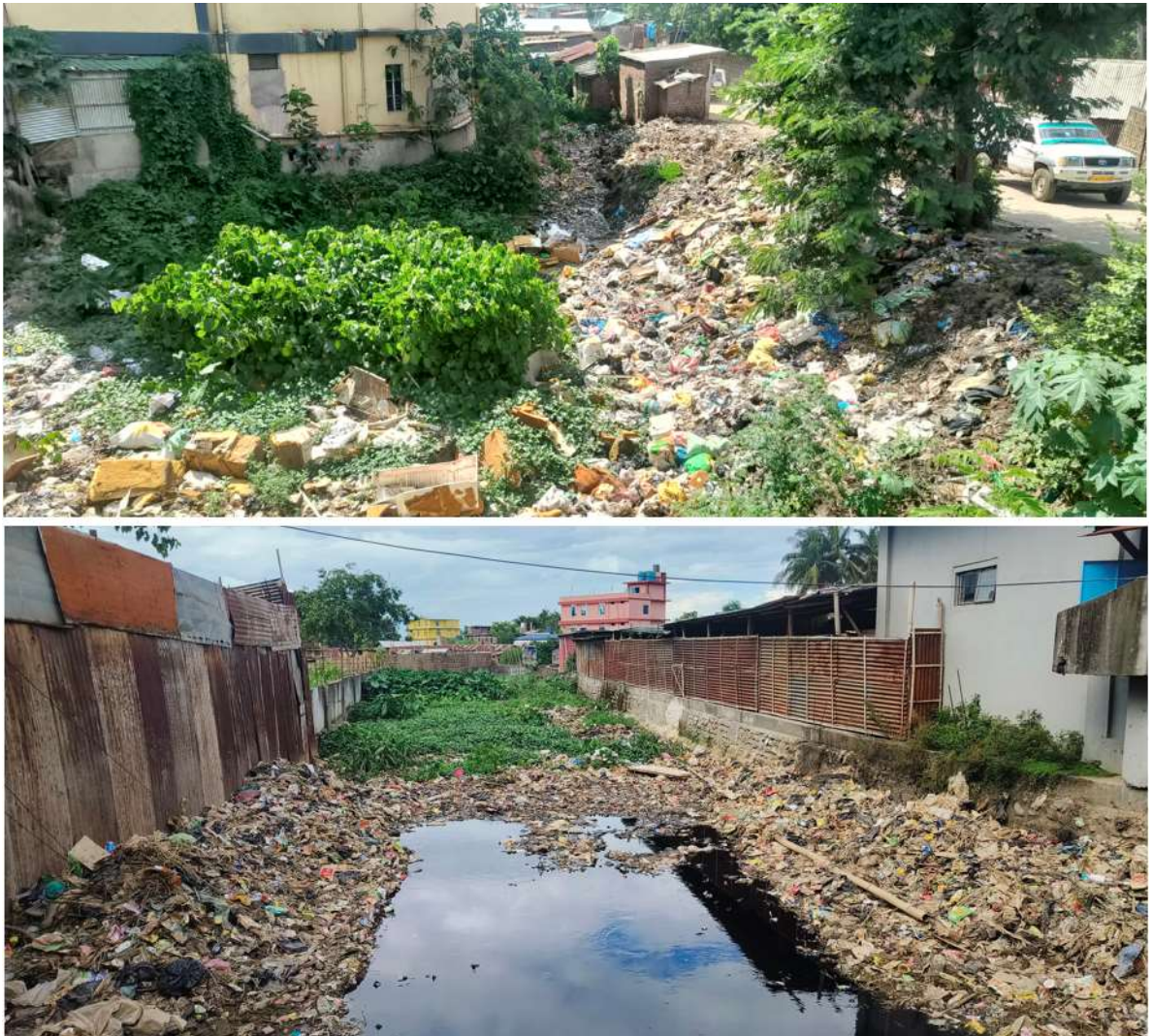
Figure 13: Pictures showing heavy garbage dumping in the drainages of Dimapur
